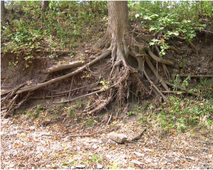
Figure 9 Trees along a stream provide multiple benefits, including increased streambank stability.
