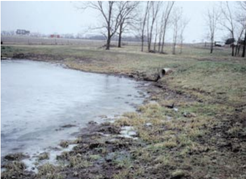
Water being held in sediment basin prior to release.
