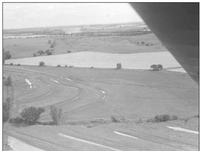
Photo 2. Poor channel drainage results in nonuniform growth and muddy spots. Defects are easy to see after a significant runoff event.
