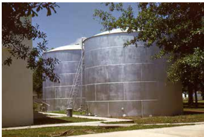
Figure 4.1. Storage tanks for fuel, feed supplements, agricultural products, and other substances may contain hazardous gases and low oxygen concentrations. (Credit: CDC Public Health Image Library)
