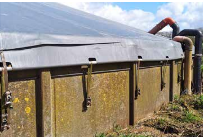
Figure 3.6. Covered above-ground manure storage tank.
