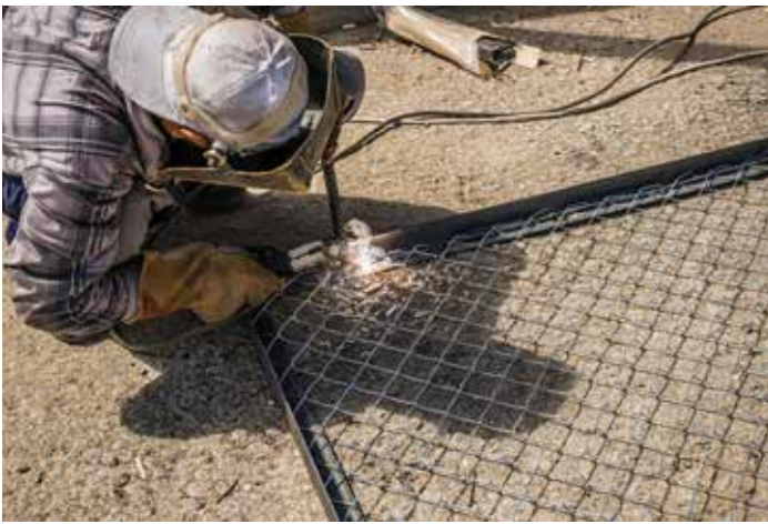
Figure 8.2. When possible, weld outdoors or in a well-ventilated area.
