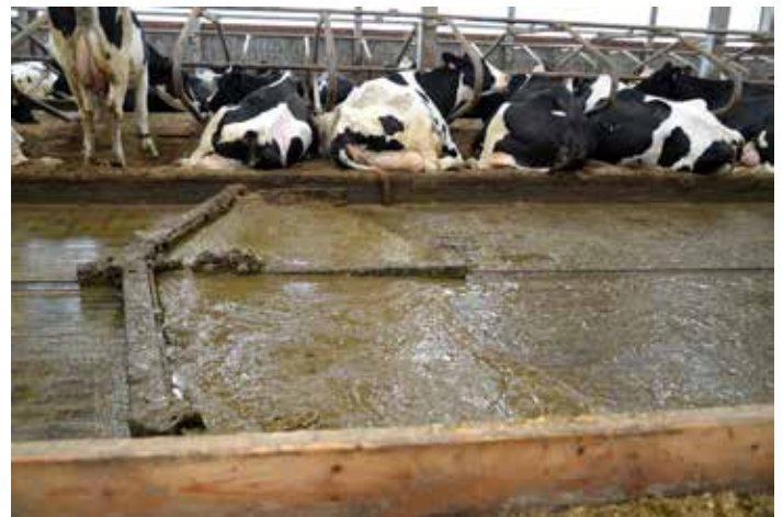
Figure 2.12. Self-cleaning floors help reduce worker exposure to manure.
