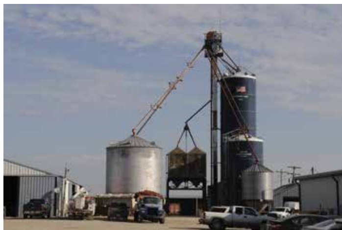
Figure 4.3. Silage storage structures may contain hazardous fermentation gases. Grain storage structures may contain fumigants.
