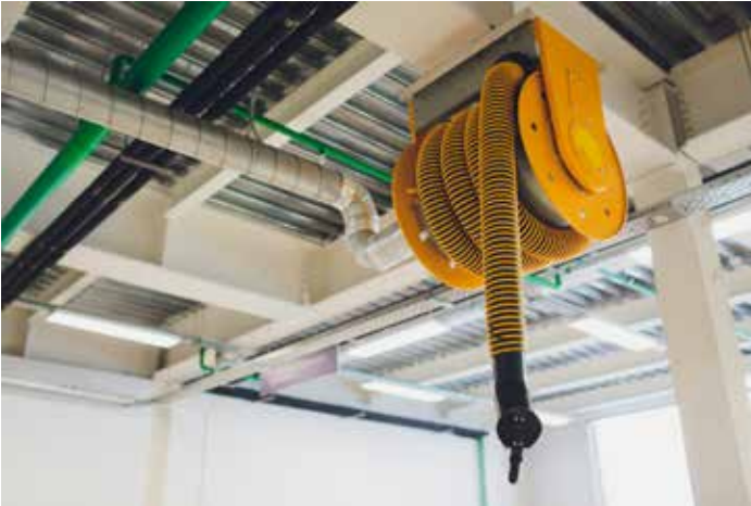
Figure 7.10. Tailpipe-exhaust extraction systems use fans and ducts to capture vehicle exhaust.
