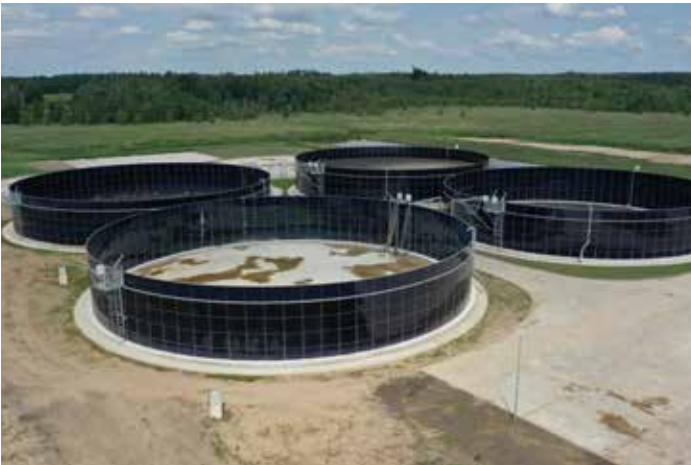
Figure 3.5. Open-air, above-ground livestock waste storage tanks.
