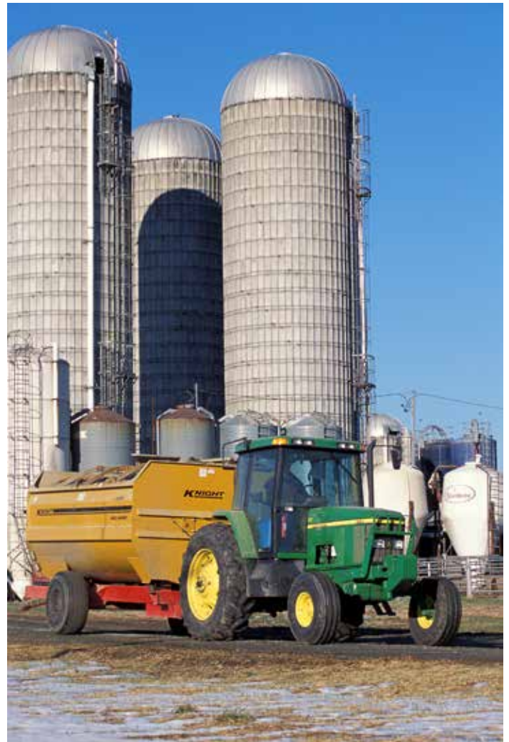
Figure 11.3. A confined space is not designed to be continuously occupied by workers. For instance, this silo was designed for storing silage and not for accommodating workers on a routine basis. (Credit: Agricultural Research Service)
