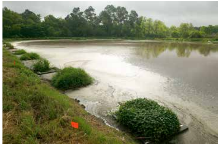
Figure 3.7. Open-air animal waste lagoon with vegetative mats to absorb nutrients. (Credit: Agricultural Research Service)
