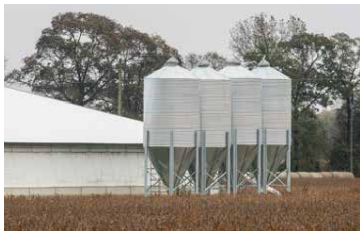
Figure 11.5. A confined space may be permit-required if it has a funnel-shaped bottom where a worker could get stuck, such as these hopper-bottom bins. (Credit: USDA)
