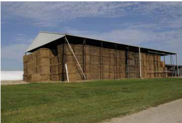
Figure 2.10. Reduce decomposition by protecting hay and straw from rain and other sources of moisture.
