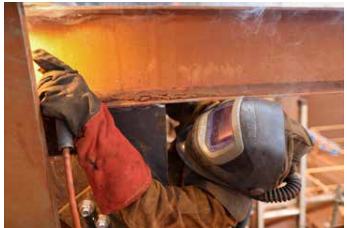
Figure 8.5. This welding helmet has a built-in powered-air-purifying respirator (PAPR) to protect the worker from fumes.
