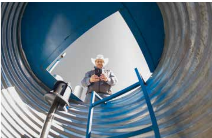
Figure 11.2. A confined space has limited means of entry and exit. To illustrate, this irrigation manhole can only be entered using the hatch and ladder. (Credit: USDA)
