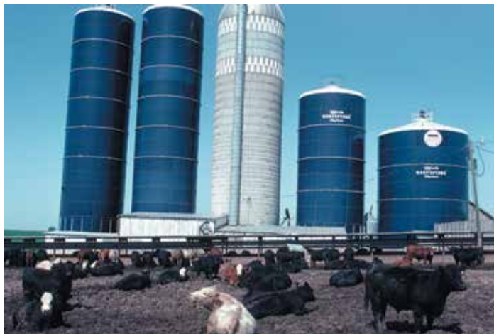
Figure 4.9. Upright oxygen-limiting silos (blue in the image) are normally loaded from the top and unloaded from the bottom. They are designed to maintain a nearly airtight environment. (Credit: Lynn Betts, USDA Natural Resources Conservation Service)
