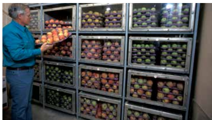
Figure 4.16. Never enter a controlled atmosphere storage room without testing the oxygen levels and following an established opening procedure. (Credit: Agricultural Research Service)
