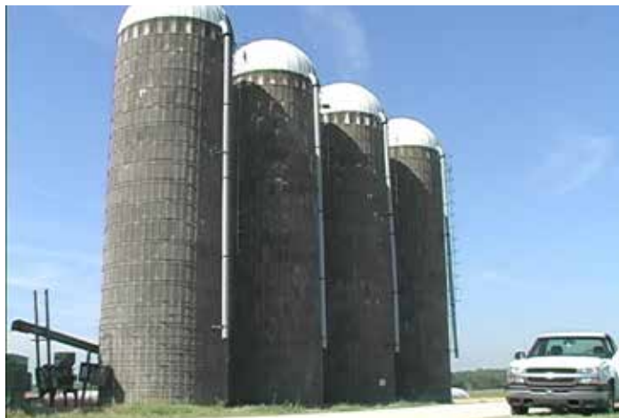
Figure 4.8. Upright concrete stave silos are usually loaded and unloaded from the top. The top may not be sealed from outside air, so a “cap” of plastic sheeting may be used to keep out as much air as possible.
