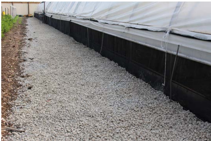
Figure 35. Gravel placed on the outside of a greenhouse to prevent weed establishment (Photo: Raymond Cloyd).
