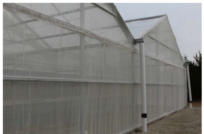
Figure 37. Insect exclusion screening placed over greenhouse opening (Photo: Raymond Cloyd).
