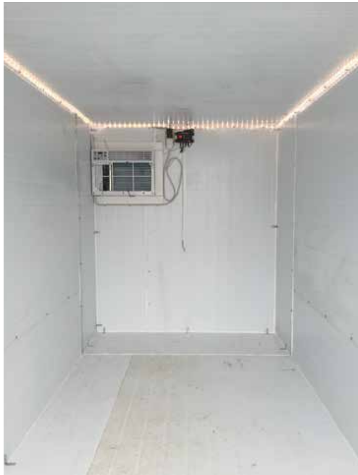
Figure 12. The trailer with cooling and lighting installed.
