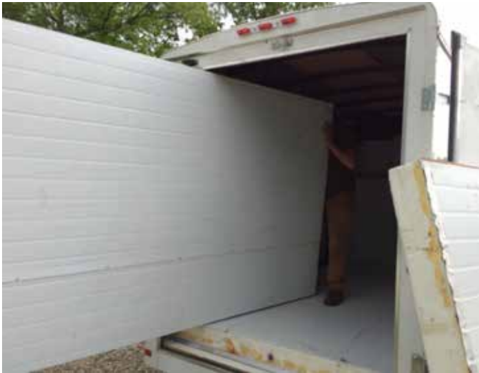
Figure 5. Assemble both side walls and check to make sure there is room to insert the ceiling panel on top.
