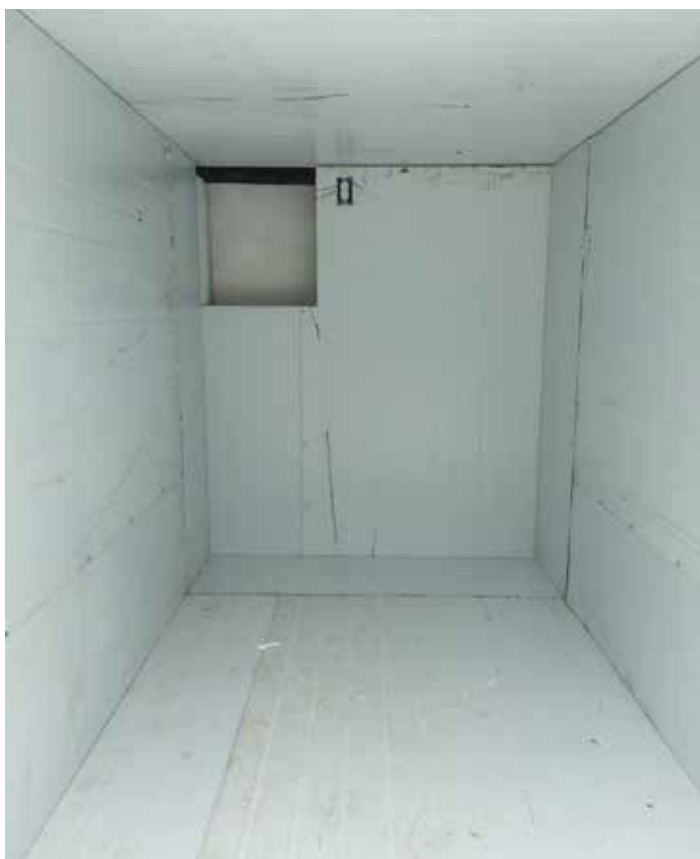
Figure 8. After installation of the insulated ceiling and wall panels.
