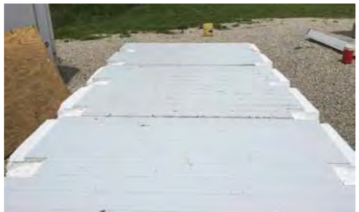
Figure 7. Notch the ceiling panel to maximize height in the trailer and avoid structural ribs that support the trailer at the corners.
