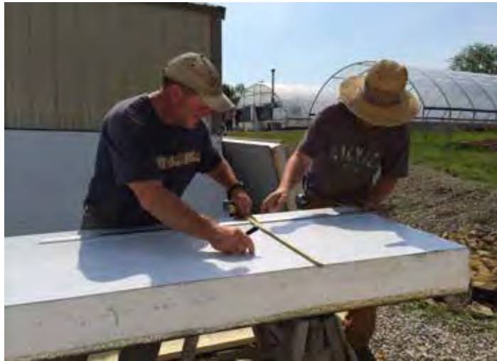
Figure 2. Measure both sides of the insulated panels before cutting the individual pieces.
